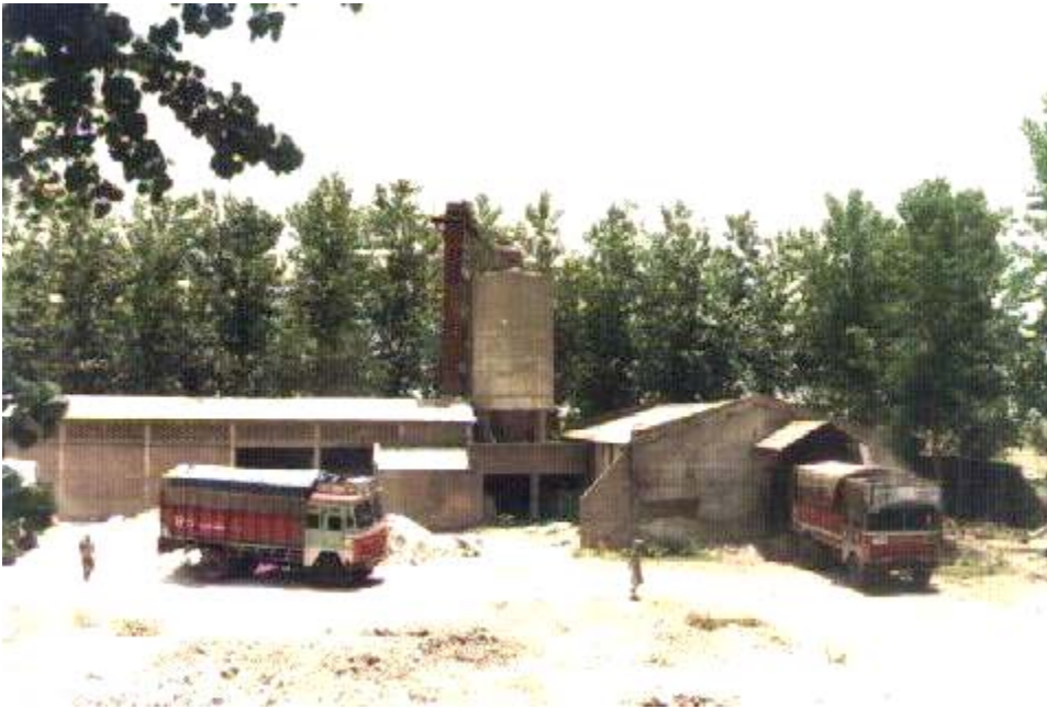
FIG 2. Cement Mill with Cement Silo, Packing Machine & Cement Godown. (This machinery that will be required if we opt for a Cement Grinding plant)
